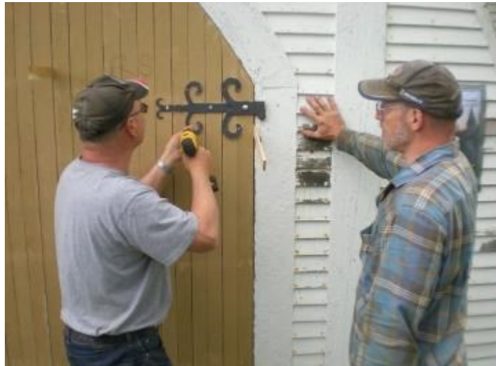
Ed Pedersen and Steven Aulis give the finishing touches to the new doors on the Canterbury Centre.
